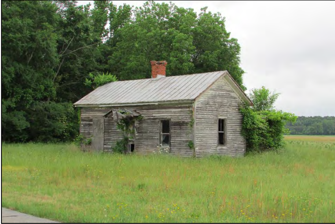
Figure 25. Mann Tenant House, front (west) and south elevations, looking northeast
