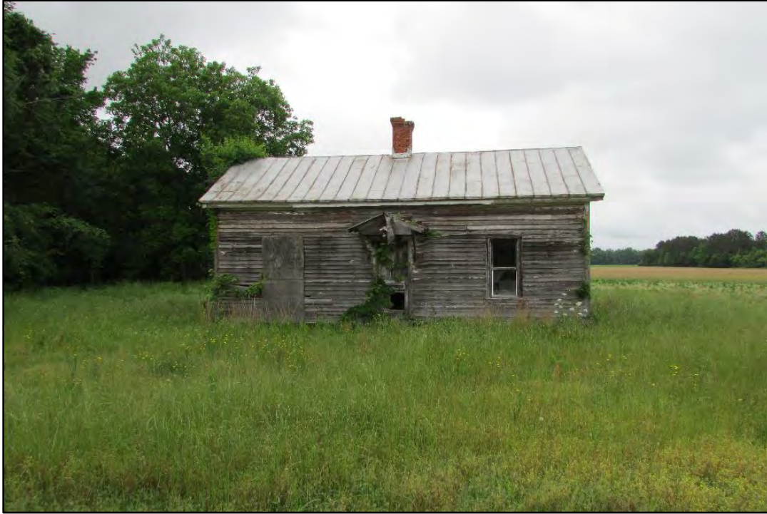
Figure 31. Mann Tenant House, front (west) façade, looking east.
