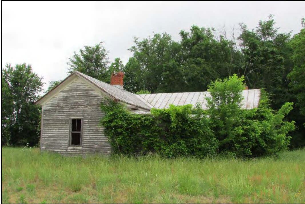
Figure 33. Mann Tenant House, south elevation, looking northwest.
