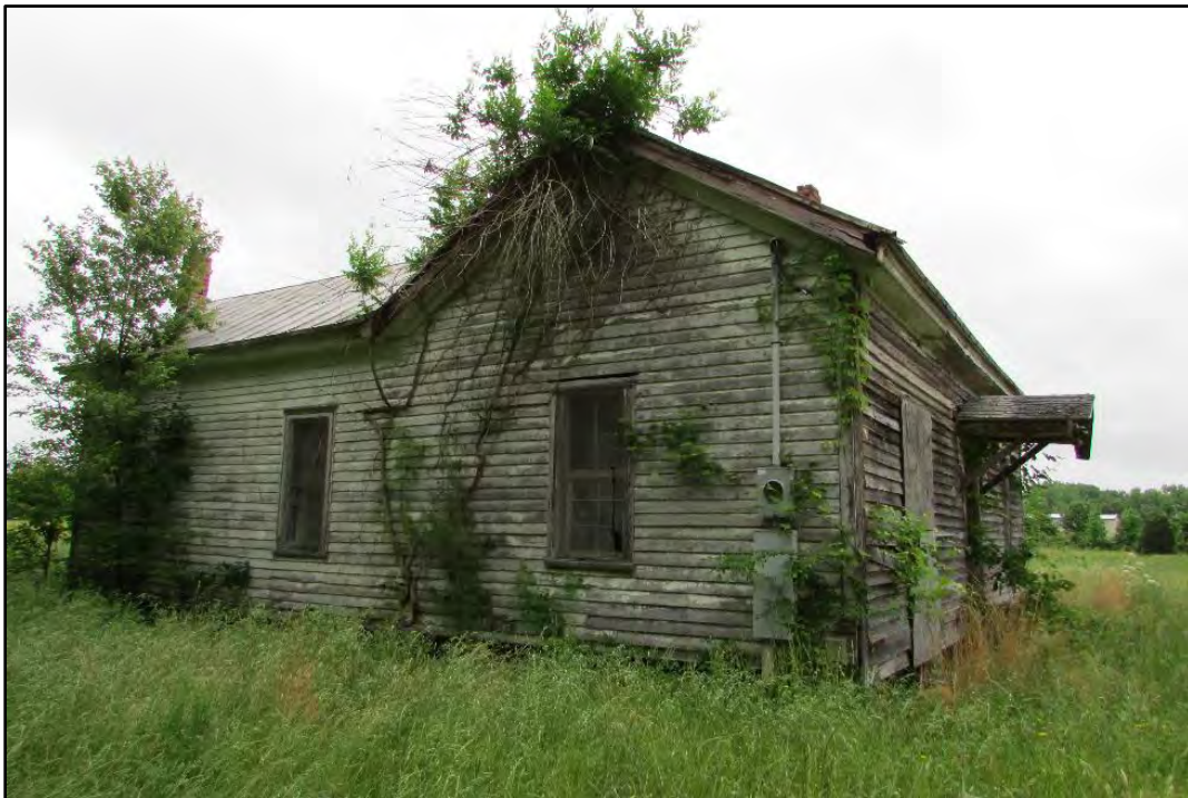
Figure 32. Mann Tenant House, north elevation, looking southeast.
