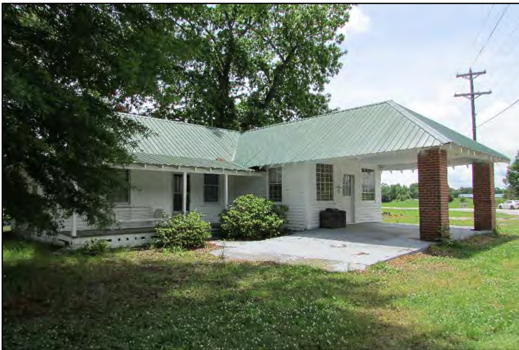
Figure 9. Moore's Store, front (northwest) elevation, looking south.
