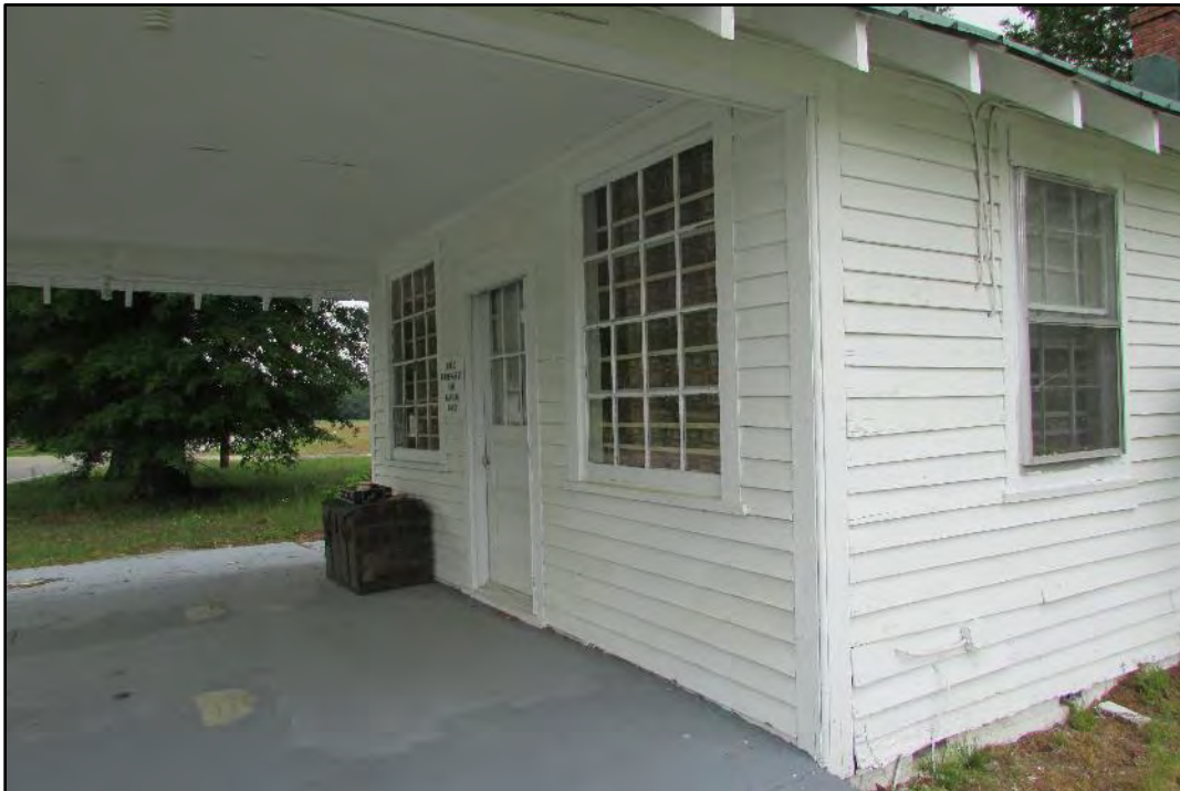
Figure 13. Moore's Store, detail of commercial façade, looking east.
