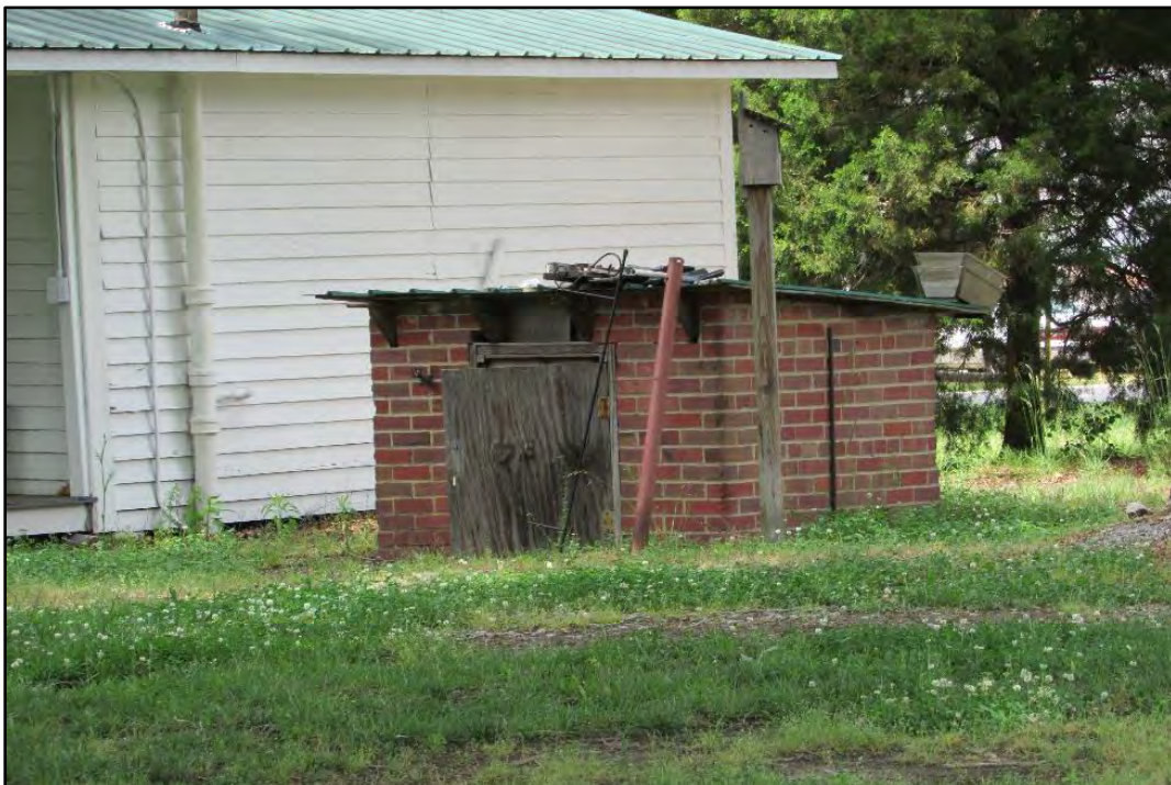
Figure 15. Pump House, looking northeast.
