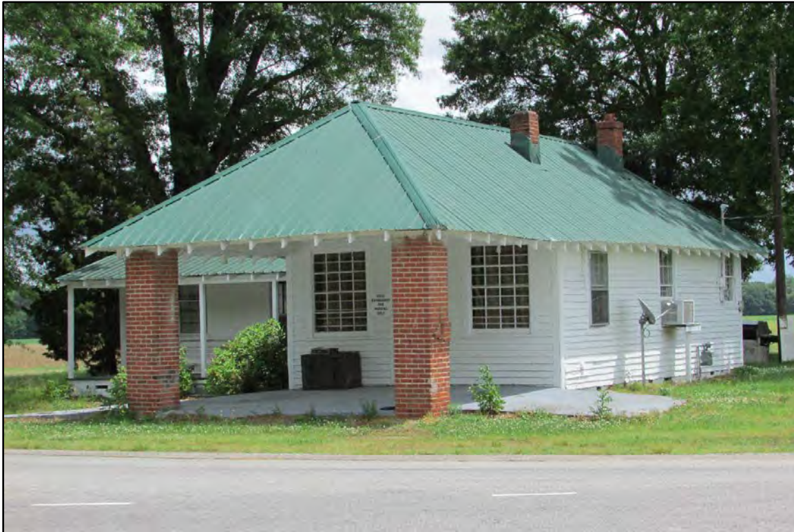
Figure 4. Moore's Store, front (northwest) elevation.
