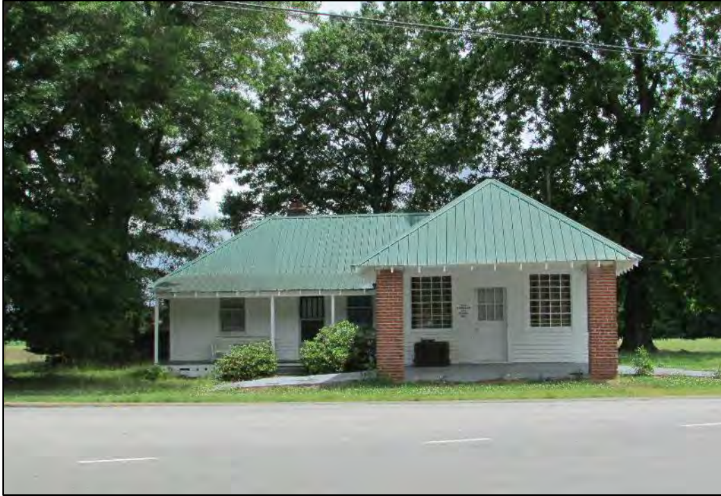
Figure 10. Moore's Store, front (northwest) elevation, looking southeast.
